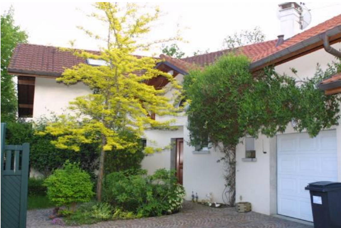
Front entrance view
